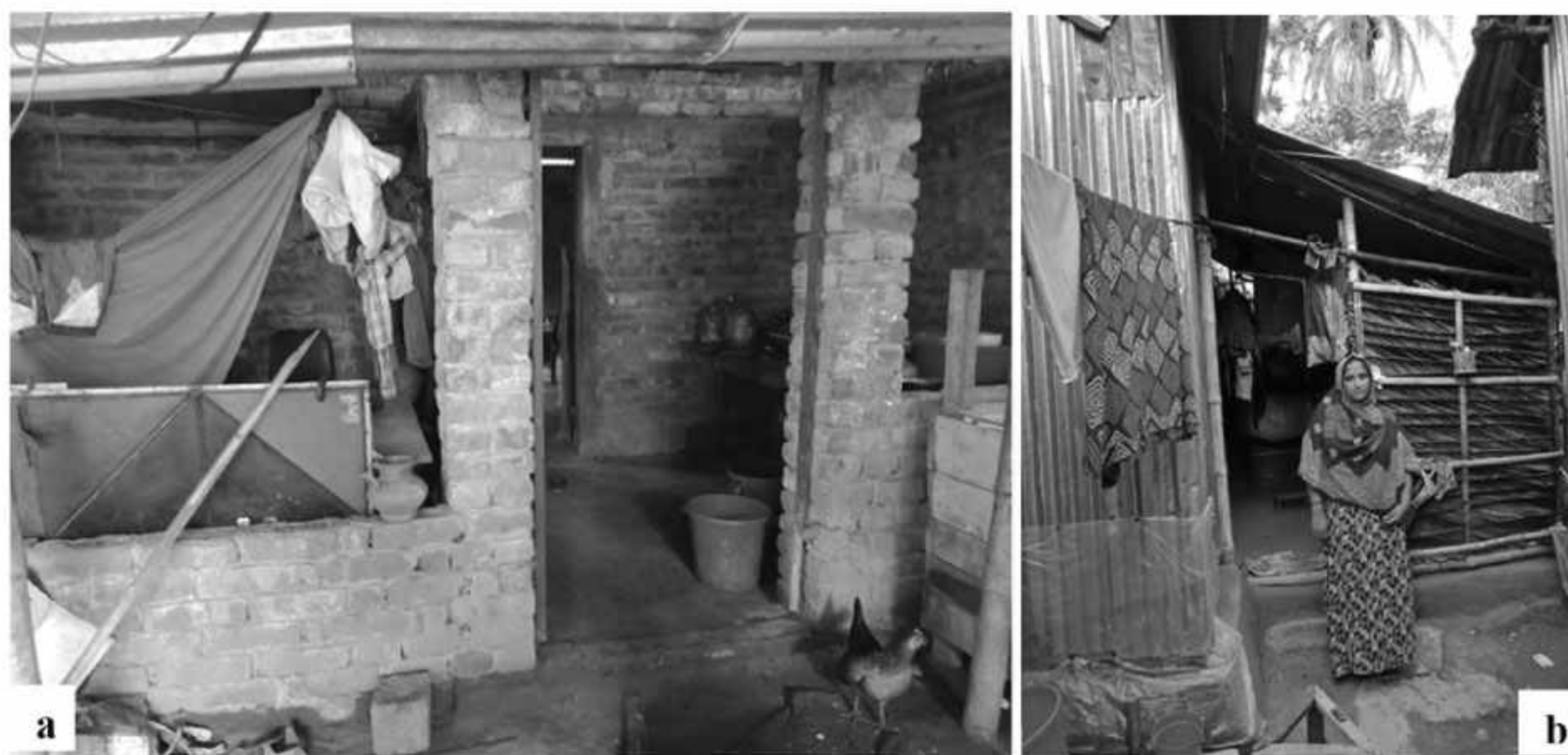
Figure 4: a) Upgradation with a new brick wall; b) Extension of kitchen and installation of new tin.
